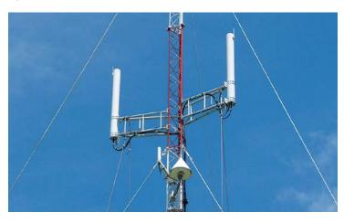
In areas with sufficient Mode A/C/S interrogation provided by local SSR or in areas with transponder overloading problems, NEO by ERA can be configurated as a fully passive solution and utilizes all available SSR replies to locate, identify and track aircraft. In this application, there is no need for additional transponder interrogation.
